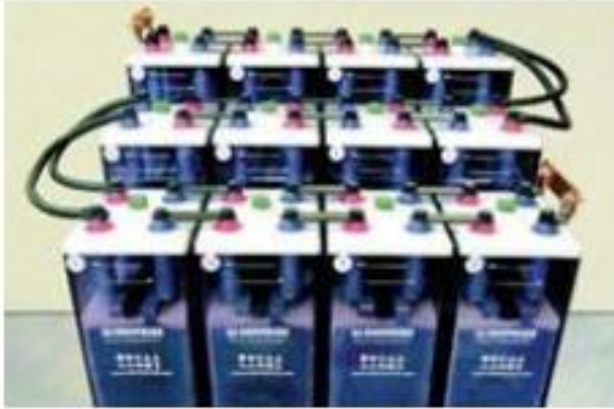
Figure 6.6.6-1 - Use of series and step connectors
