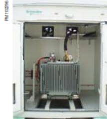
Transformer in PV box
